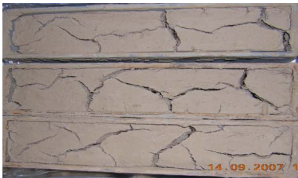
Figure 4. Shrinkage and crack formation for clay plaster.
